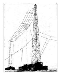
Multiwire <u>T</u> antenna of radio station WBZ, Massachusetts, USA, 1925. T antennas were the first antennas used for medium wave broadcasting, and are still used at lower power.
